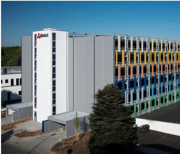
Completed multi-storey car park
